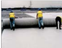
Finesse Pozidrain - typical landfill drainage and gas venting
