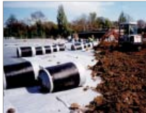
Buried reservoir drainage with Finesse Deckdrain
