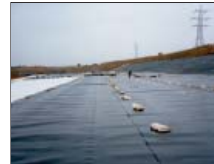
Landfill lining with Finesse Alphasine
