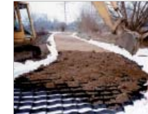
Access road with Erosoweb
