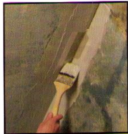
5) Over-paint with Aquaproof Compound
