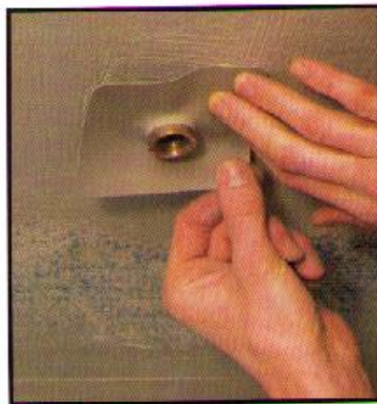
3) Apply pipe inlet/outlet details
