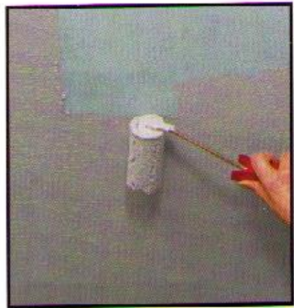
6) Apply 2 coats Aquaproof Compound
